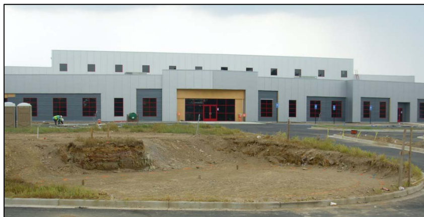
Construction of Rausch & Pausch, L.P. Facility in Auburn
